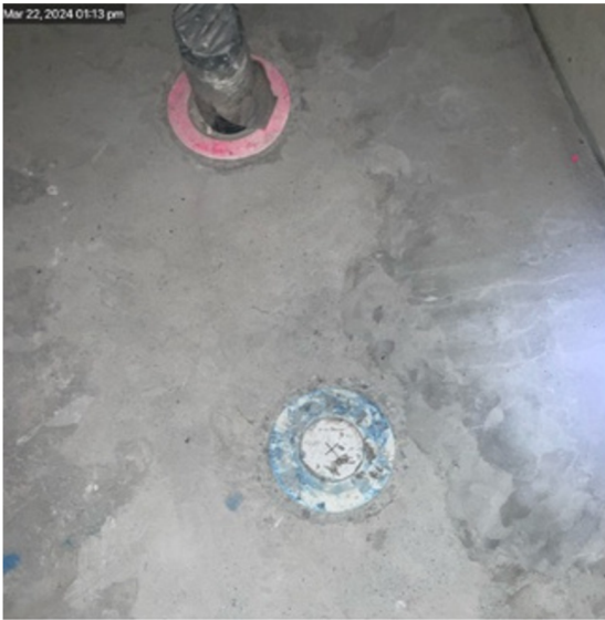
Puddle Flanges installed Flush into screed. Membrane installed above screed
