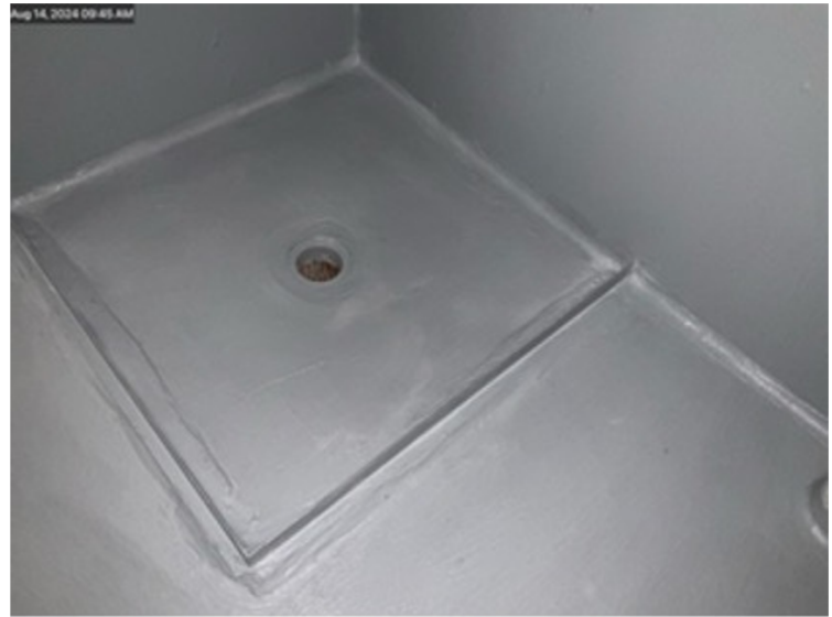
Puddle Flanges installed Flush into screed. Membrane installed above screed
